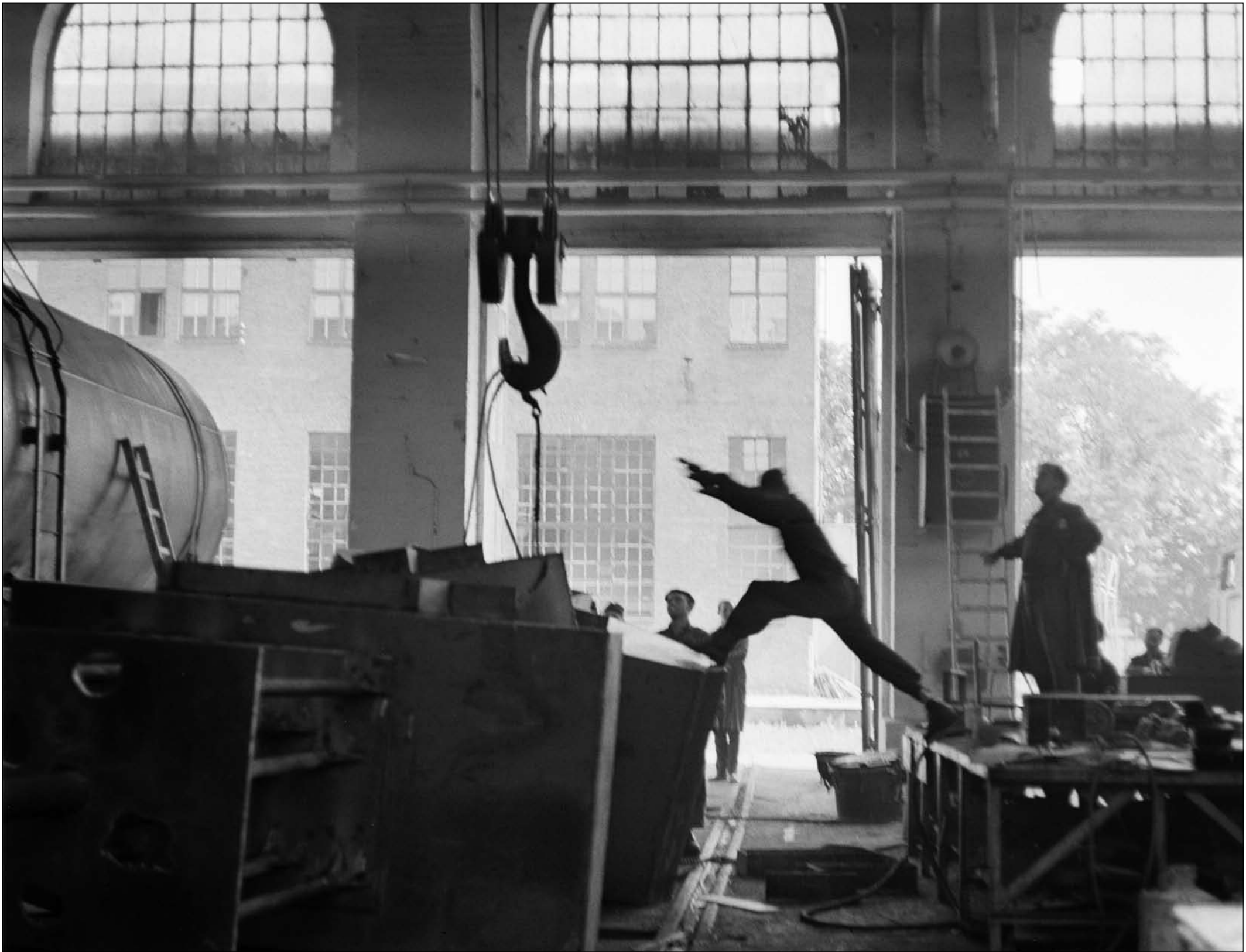
Bogdan Łopieński, picture story from the 1st Biennale of Spatial Forms in Elbląg, 1965. A spatial form by Andrzej Matuszewski being lifted.
