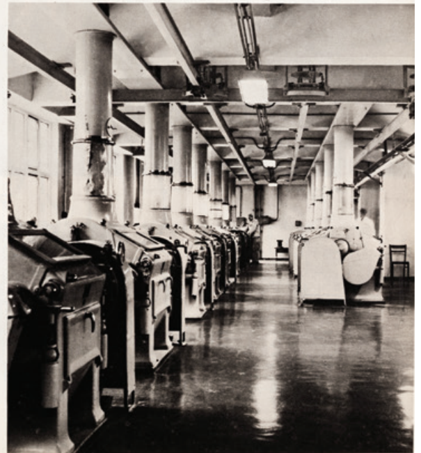
Roller grain milling machines
